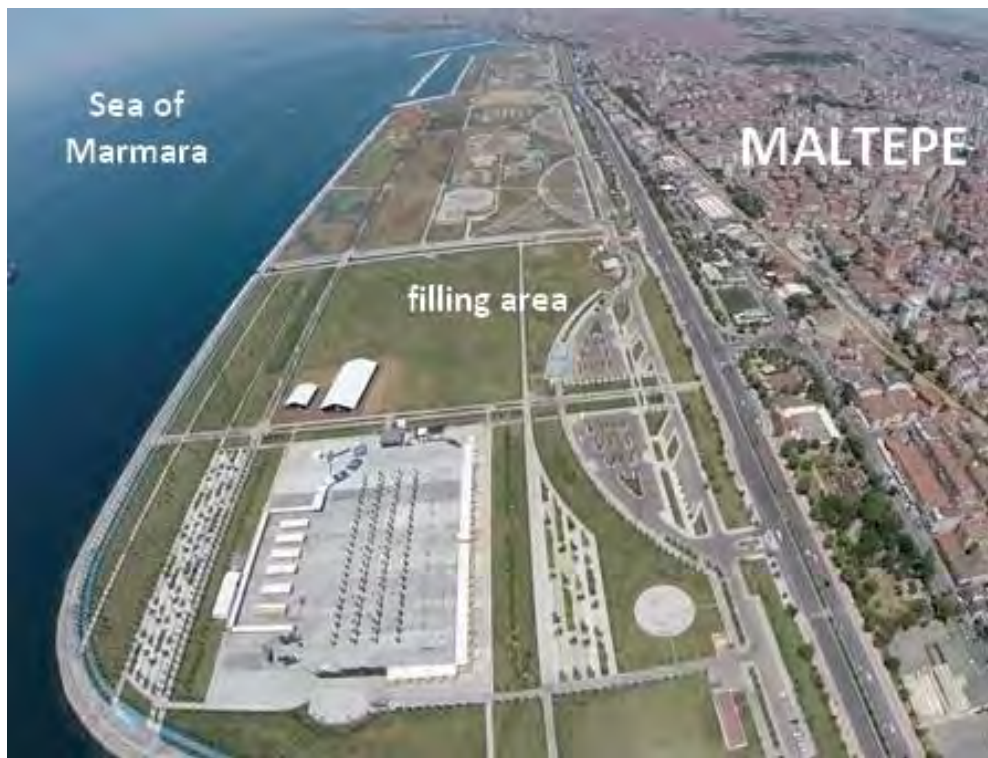
Photo 1. Maltepe fillings along the Sea of Marmara shores in Anatolian part of İstanbul ( http://www.milliyet.com.tr/gundem/dev-park-havadan-goruntulendi-1911144/son-dakikagundem/SonDakikaGaleri/13.07.2014/1911144/default.htm?PAGE=2 ).
